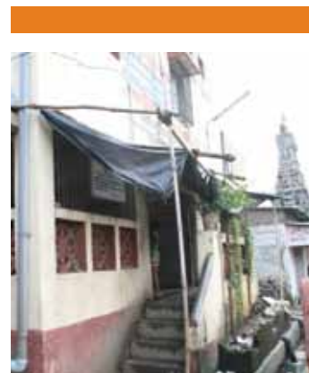
Toilet Block 10 was constructed in 2007 under the Mumbai Sewage Disposal Project
