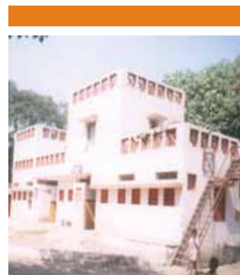
A toilet block in Mumbai with a caretaker room at the top
