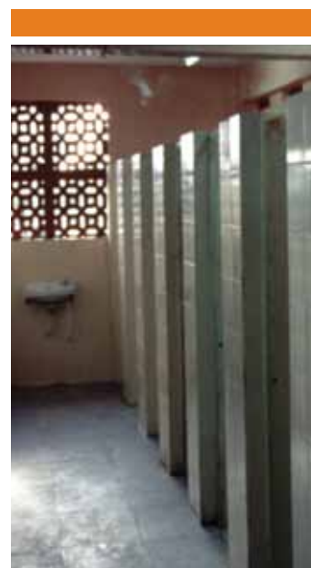
Interior of a community toilet block
