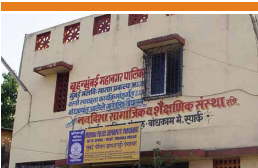
A toilet block constructed in 2003 by SPARC under the Slum Sanitation Program of the Mumbai Sewerage Disposal Project funded by the World Bank
